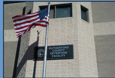
Rutherford County Detention Center
