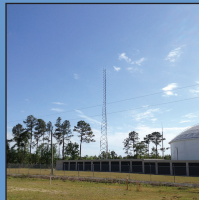
152' Rohn Self-Supported Tower Constructed by DoubleRadius
