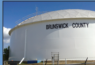
Brunswick County Public Water Storage Tank
