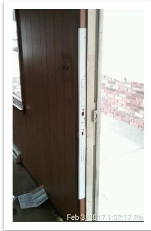
Photo shows door jamb protection product being installed.
