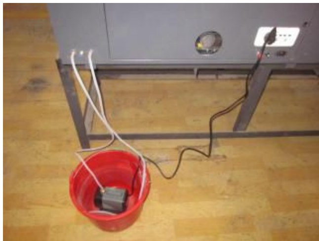
Picture 11 Water Pump Installation
