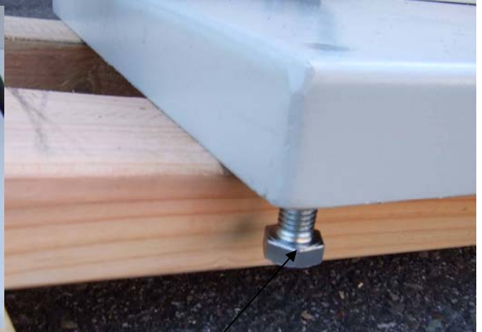
Levelling bolt
